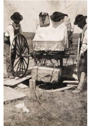
500 lb stone being lowered for Brown Valley Base. 98th Meridian survey. Jasper Bilby on the right. Circa 1903
