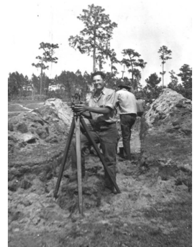
CCC land surveyor, Clyde Kerce Highlands County
